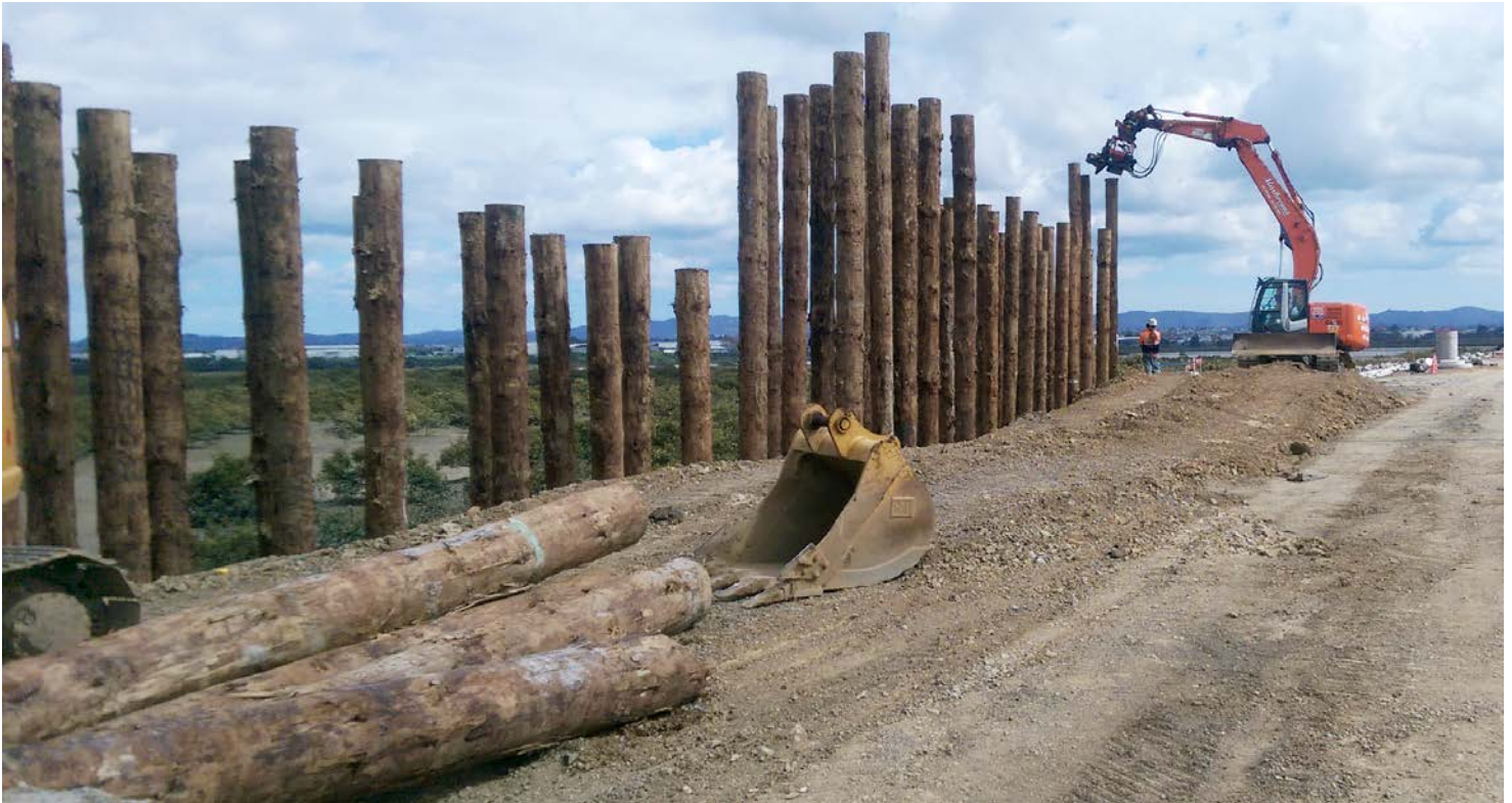
Causeway Upgrade project, SH 16 Motorway, Auckland, NZ
